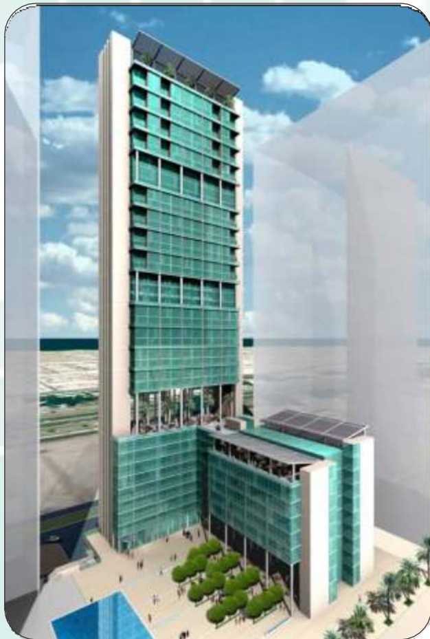
LIBERTY HOUSE TOWER ON PLOT NO-CP-01 AT DIFC, DUBAI.
