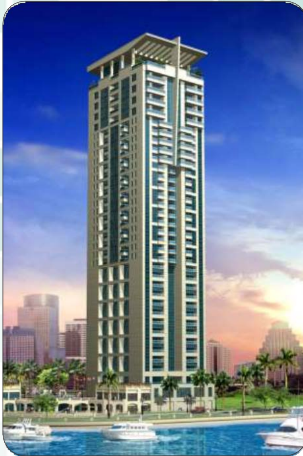
PALLADIUM TOWER ON PLOT NO C3 AT JUMEIRAH LAKE TOWERS, DUBAI. (3B+G34 FLOORS)
